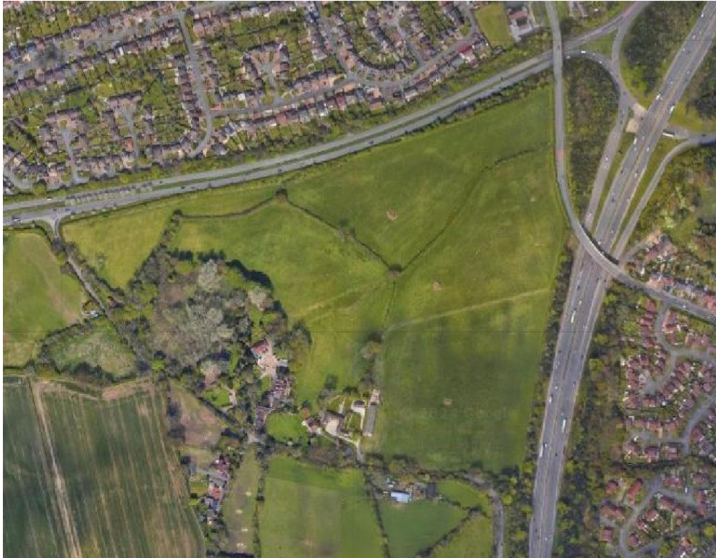
Aerial Photograph showing the Site and its immediate context
