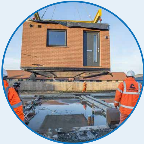
Housing being erected on site using MMC pre-fabrication methods (Source: building.co.uk)
