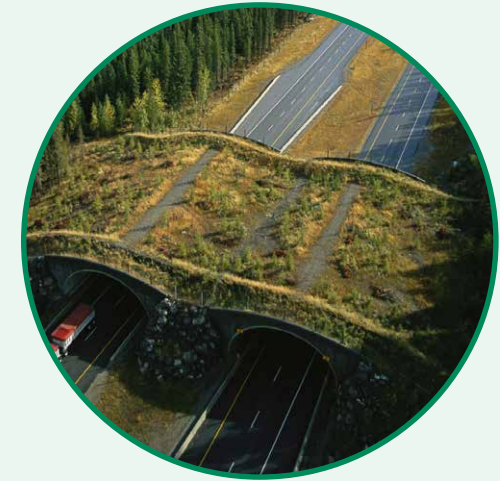
An example of a Biodiversity Corridor Bridge over a main road. (Source: Pintrest)
