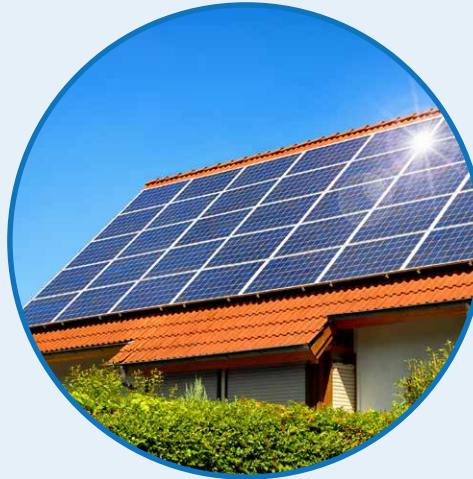
PV Solar Panels (Source: Energy Saving Trust)
