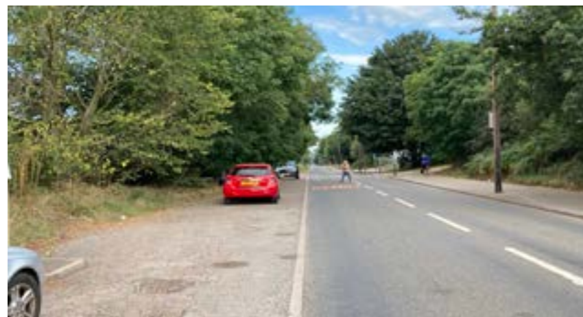
Ad hoc parking on verge and no formal crossing points are safety issue
