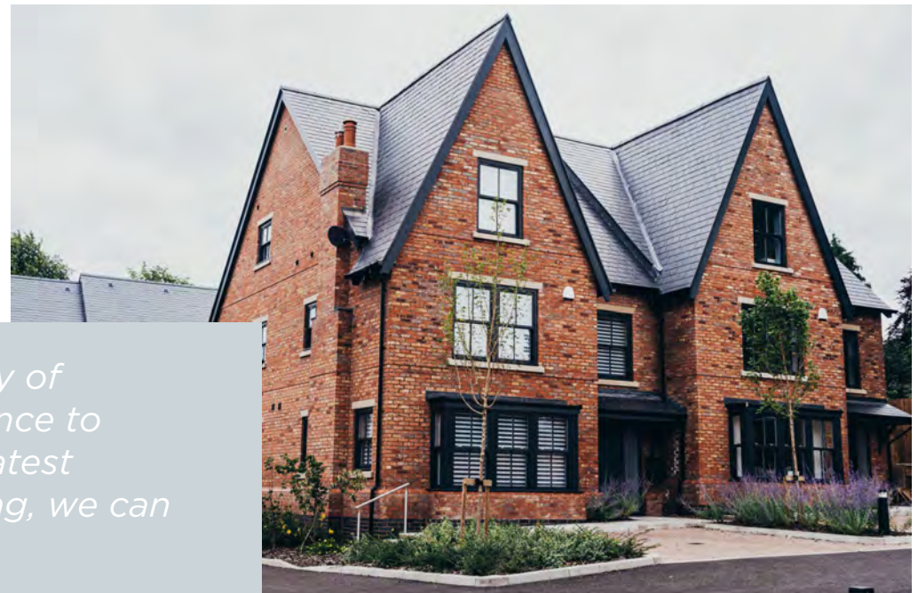
Above: Interiors of St Georges Townhouse Development, Below: Homes at Oaklands
